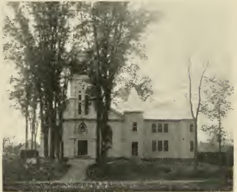
CONGREGATIONAL CHURCH. Remodeled 1898.
